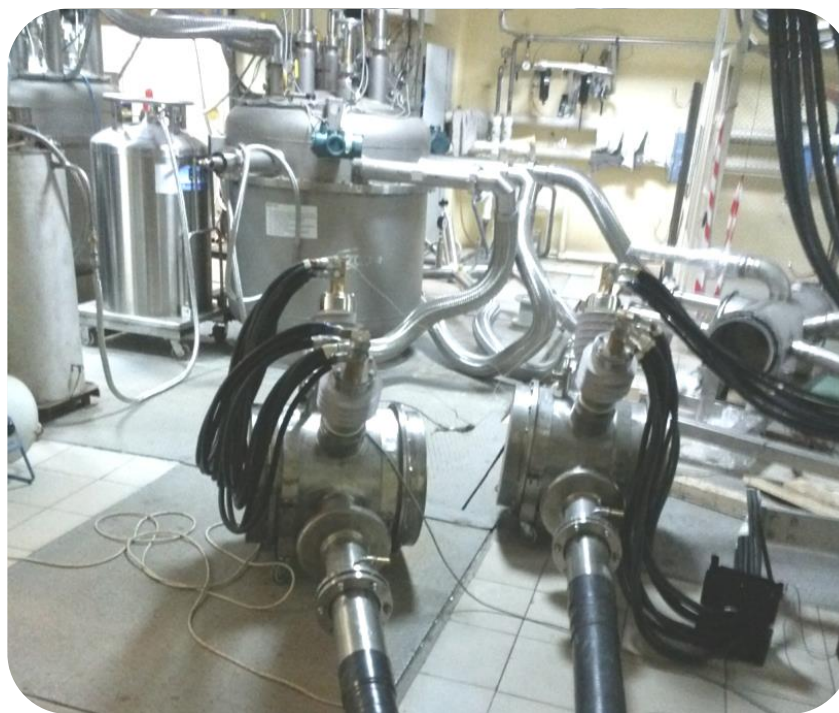
Connection of the HTS cable to the Cryogenic System
