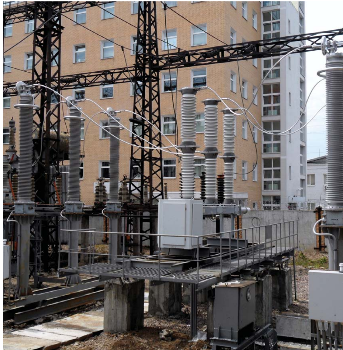
The optical transformers of the Digital Substation Test Site in R&D Center at FGC UES
