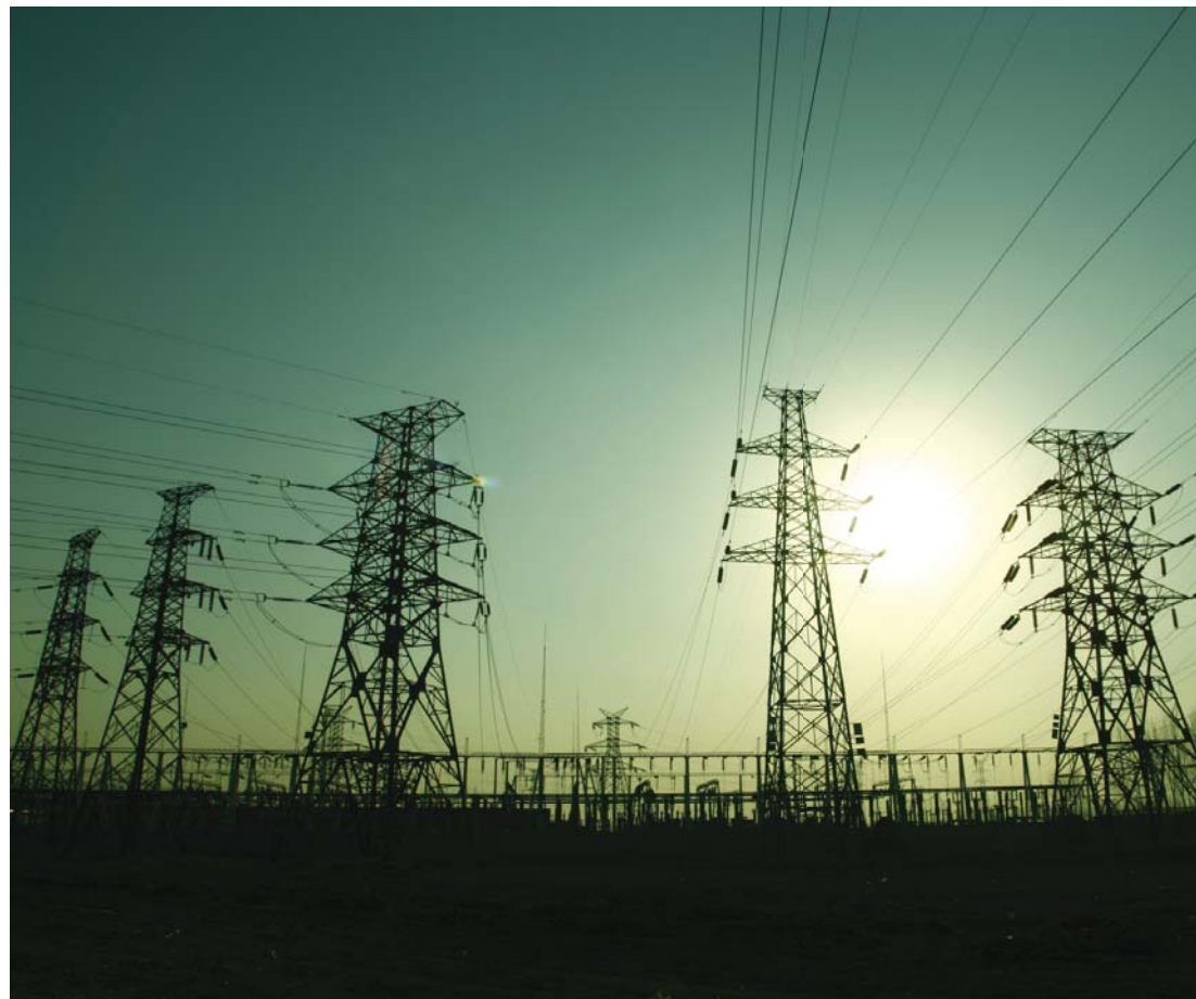
Series capacitive compensation devices provide capacity increase of the extended power transmission lines
