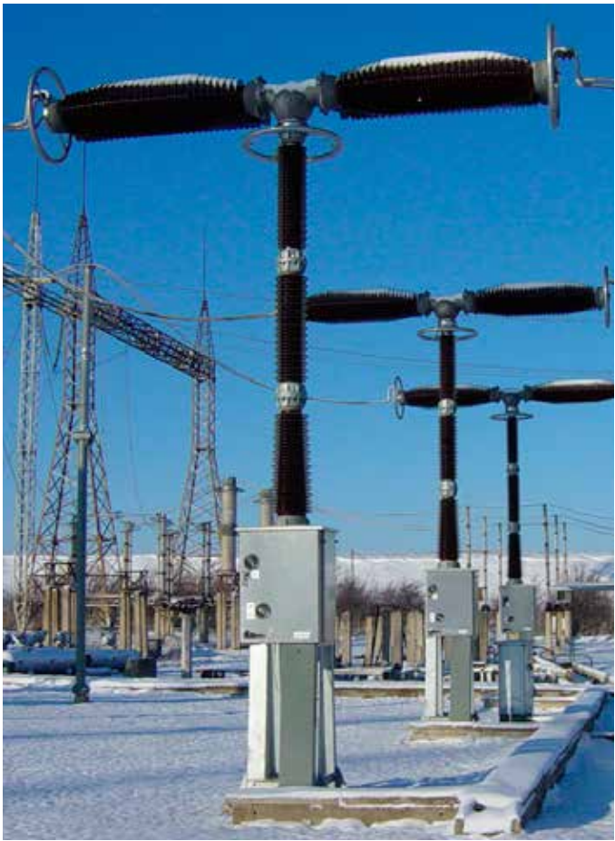
Fig. 2. Live tank SF 6 circuit-breaker. For low temperature use, it is filled with gas mixture
