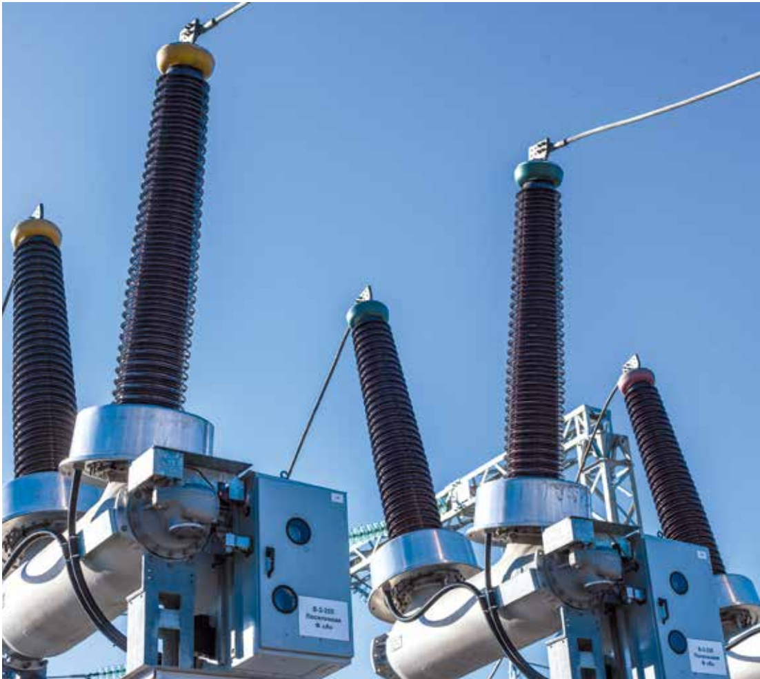
Since the early 80s, SF 6 circuit-breakers became widely used in 6-220 kV voltage class electric power systems
