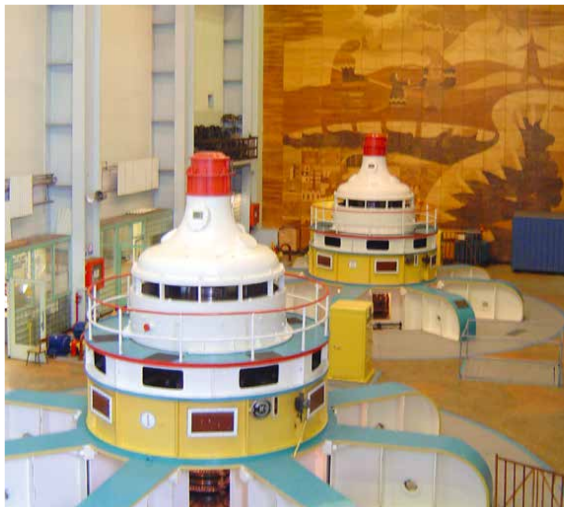
Power house of the Yovskaya hydroelectric power plant (Murmansk region)
